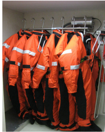
wall-mounted drying system for clothing
